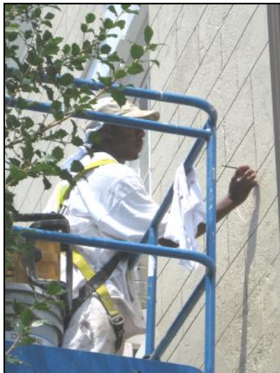
Sobrinski Painting employee uses a small paintbrush to detail the blocks on the Stroud Mansion.
