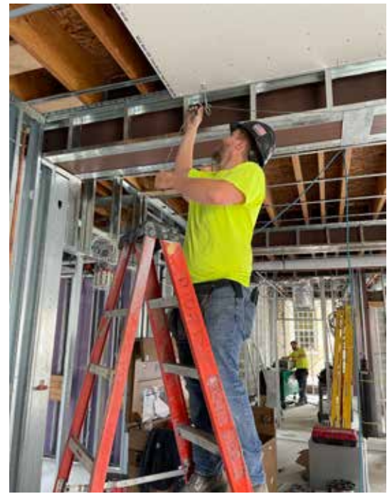
Lots going on inside the addition as well.
