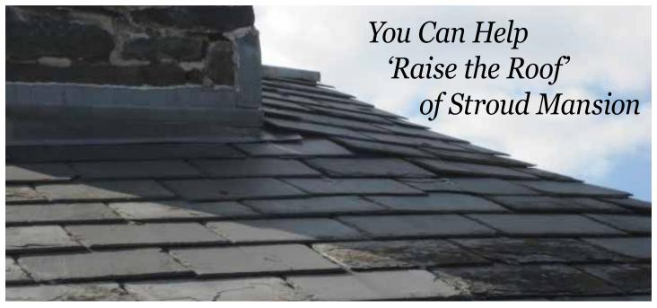
\$110,000 project: Replacing the roof on the Stroud Mansion. Notice the deterioration of the slate and the sagging roofline.
